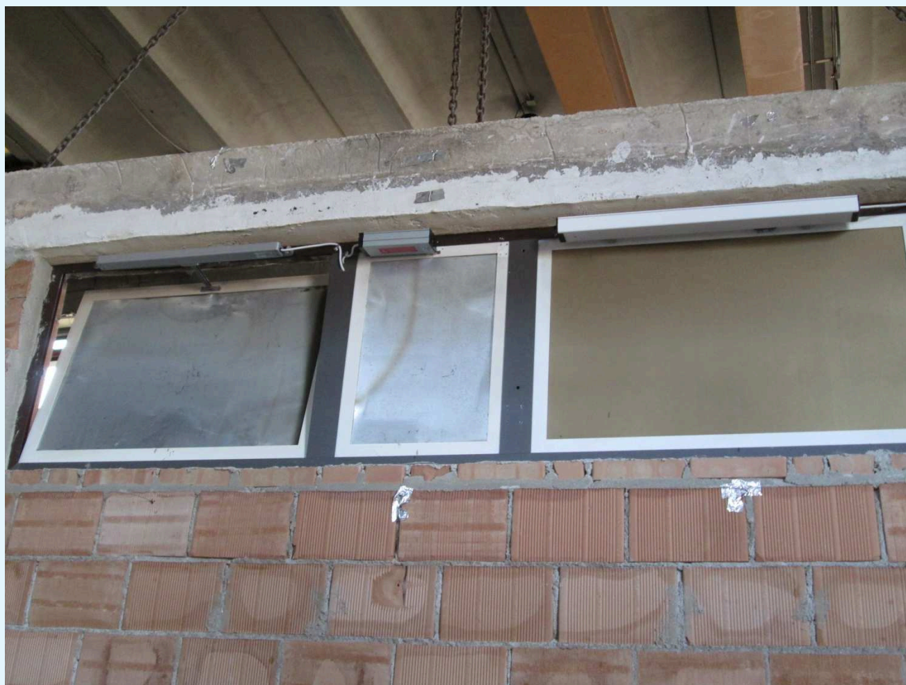
Photo of masonry with ventilators (internal view)
