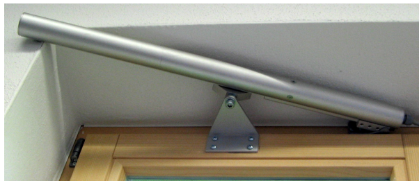
Figure 7: Mounting example with ZVE-UNI
